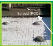
Slope for water drainage
