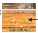
CONCRETE / SOIL FOR 1"/10' GRADIENT
