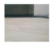
BUILDING ELEMENT Plaster over grouted brick tiles for terrace finishing.
