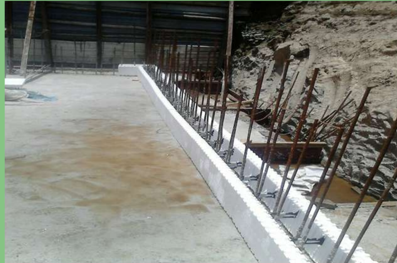
Raft Foundation for basement with double layer steel
