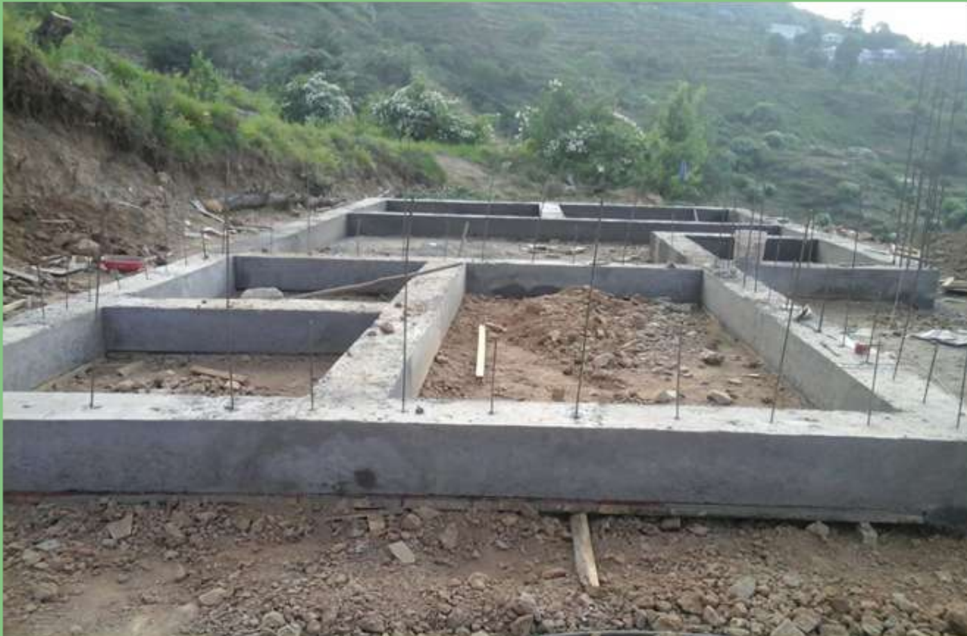
Strip Foundation / Plinth beam with starting steel
