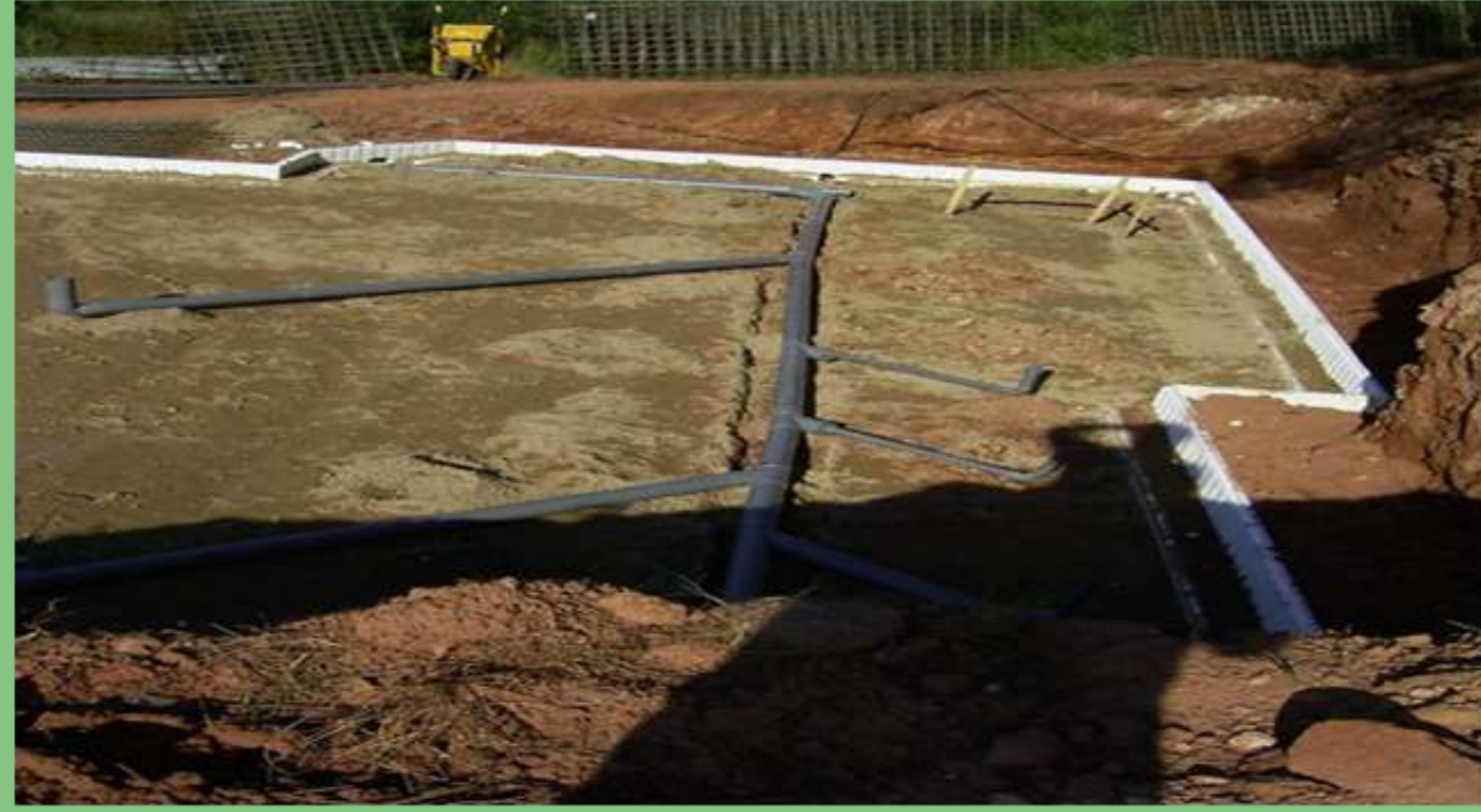
Sewage Pipeline Network
